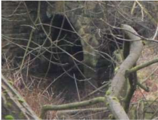
The Cockey Moor Culvert at the river Irwell
