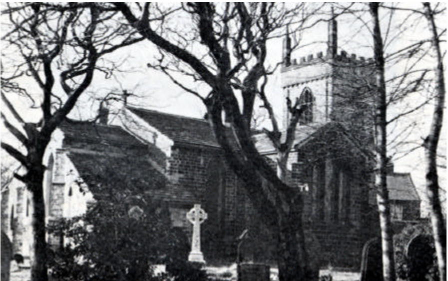
The north side of the Church
