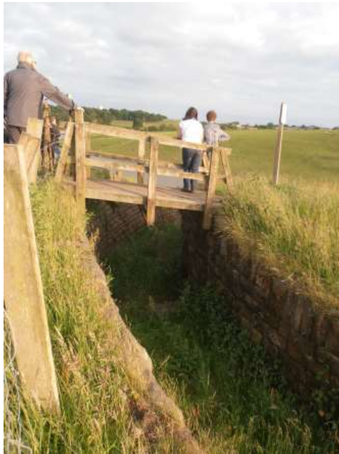
Bridge across the overflow between the lodges
